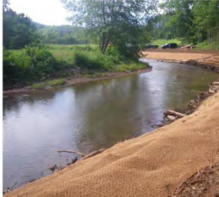
**Before and after photos of a bend in the creek. The failure of the bank was repaired with a rock vane on the inside of the curve and geolift and bank sloping on the outside.**
