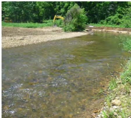
**Before and after photos of the mid-channel. The build-up of a bar was corrected with a rock vane and a shifting of the channel.**
